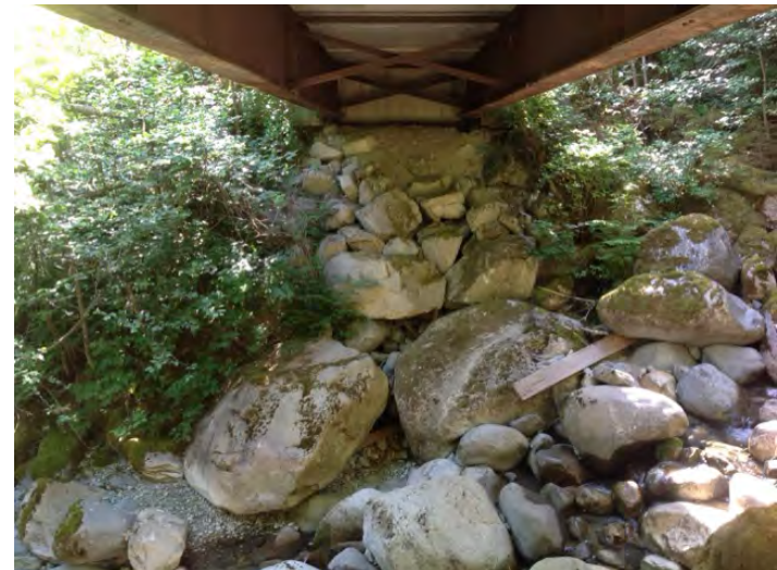
Right Bank Abutment when facing downstream
