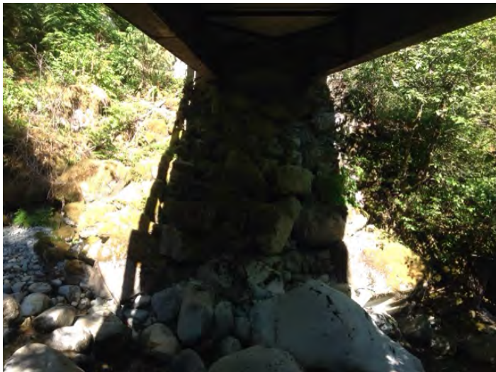
Left Bank Abutment when facing downstream
